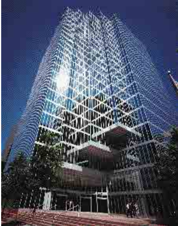
PROJECT: Canadian Imperial Bank of Commerce, Vancouver, B.C. ARCHITECT: Musson, Cattell, Mackey, Partnership CONS. ENGINEER: Domco
