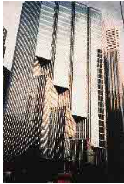
PROJECT: Sun Life Centre, Toronto, ONT. ARCHITECT: The Webb, Zerala, Menkes, Housden Partnership CONS. ENGINEER: Mulvey & Banani International Inc.
