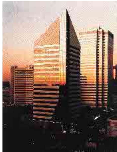
PROJECT: IPL Building, Edmonton, ALTA. ARCHITECT: WayneScott CONS. ENGINEER: Wasnea and Beaubien
