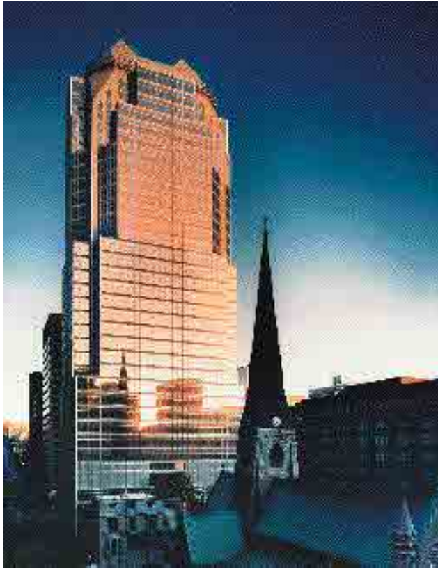
PROJECT: La Maison des Cooperants, Montreal, Que. ARCHITECT: Webb, Zerala, Menkes, Housden CONS. ENGINEER: Les Consultants C.R.S.Inc.
